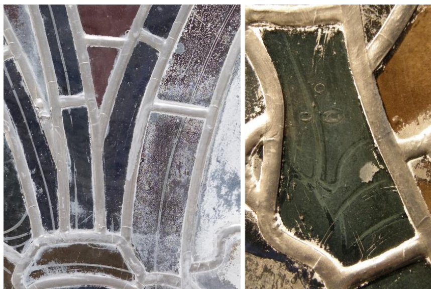
Fig. 3. Berne Minster, preparatory tracings on the reverse of the Passion (I, 5c) and the Ten Thousand Knights window (I, 4c, see also fig. 2). Some of the tracings are preserved as entire brushstrokes, while from others only parallel outlines remain, and even these are often confined to marginal areas. © Stefan Trümpler.
